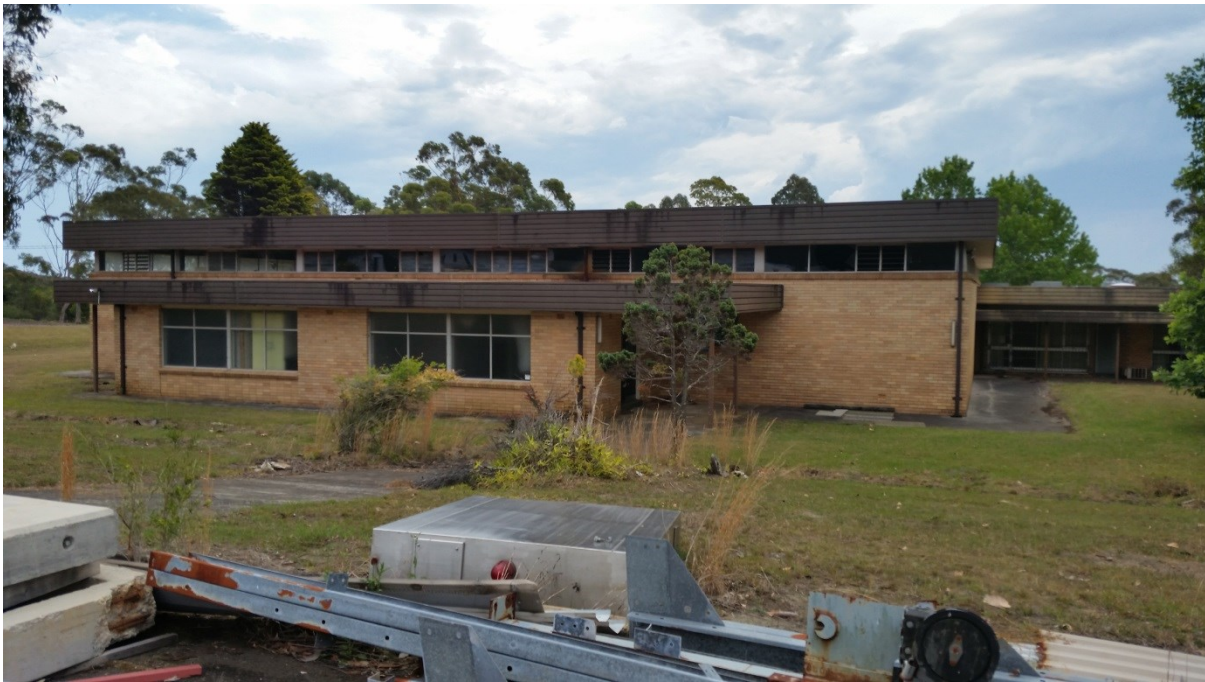
4. Former administration building and shower block
