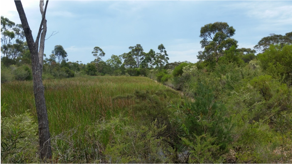
7. Former effluent lagoons
