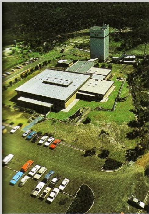
Darkes Forest Mine Surface Facilities, 1972
